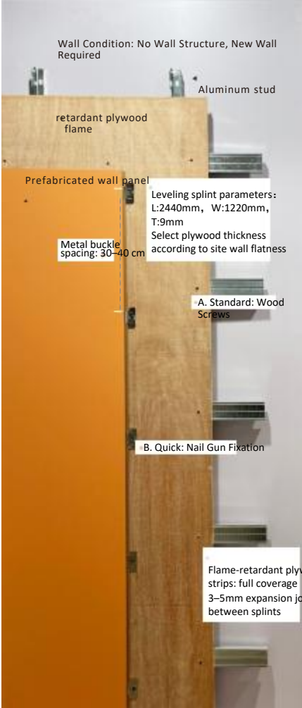
Situation 3 Wood clamping board installation
